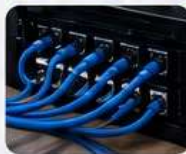
STRUCTURED CABLE INSTALLATION
